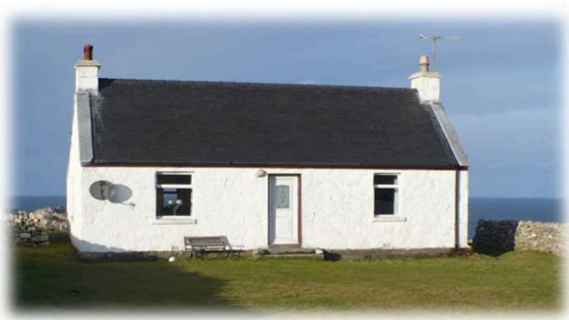
Figure 12: Nearest neighbour Benmeanach cottage has the similar width and height
